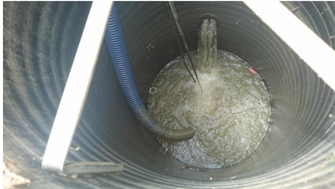
Pumping away groundwater to lower groundwater level
